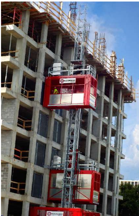
Construction Hoists
